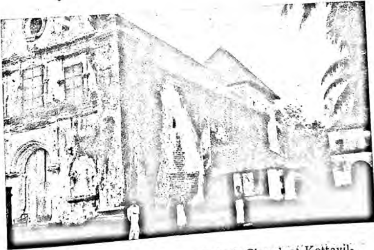
21. A view of the old Roman Catholic Church at Kottayil-Kovilakam in Chennamangalam, built by the Jesuit Fathers in the 16th century A. D. or earlier.
