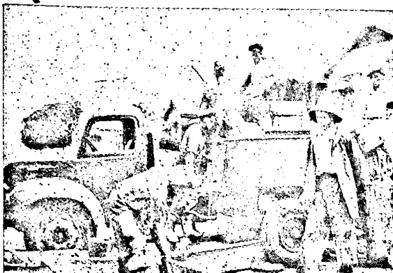
Plate 21 —The mortar-mixer unit fitted on a motor truck; sand and water being added on volumetric basis.
